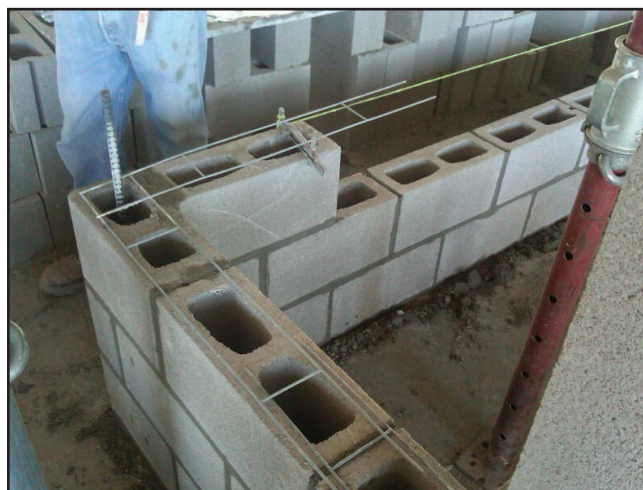
Figure 4 - Ladder type joint reinforcement laid dry on the masonry units
