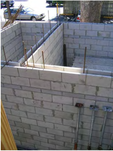
bond beam using intel block
