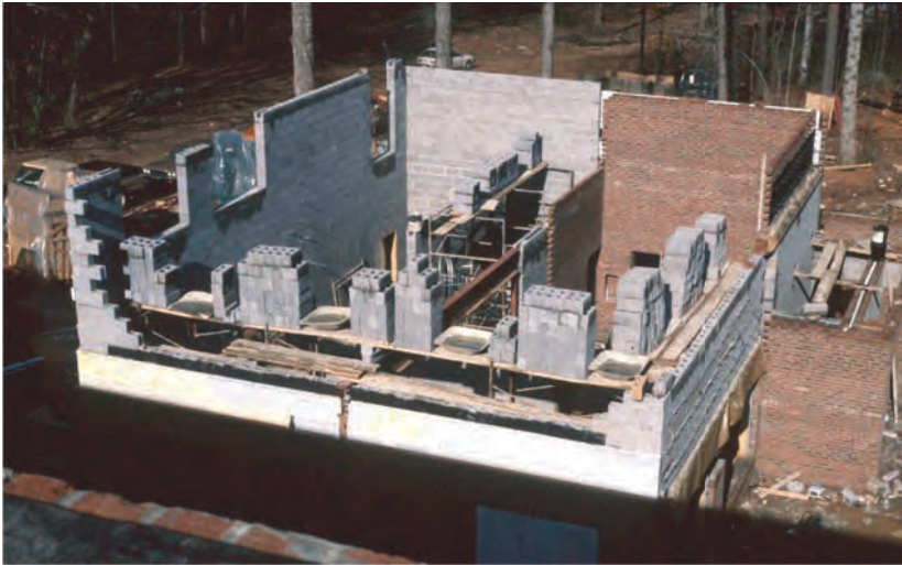
REINFORCED CONCRETE BLOCK WALLS When concrete block walls are subjected to lateral forces such as caused by wind, earth pressure below grade, and earthquakes, they may be reinforced as illustrated above.
