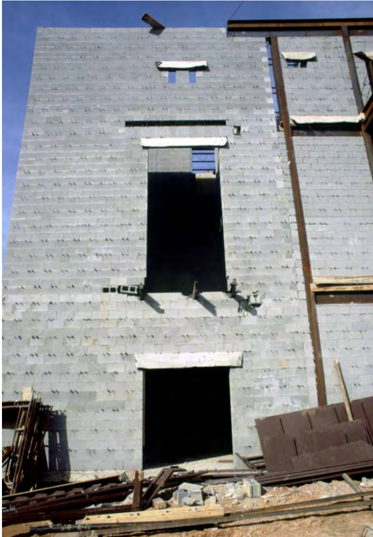
Attempting to maintain plumb cladding on an out-of-plumb frame can lead to a range of problems.
