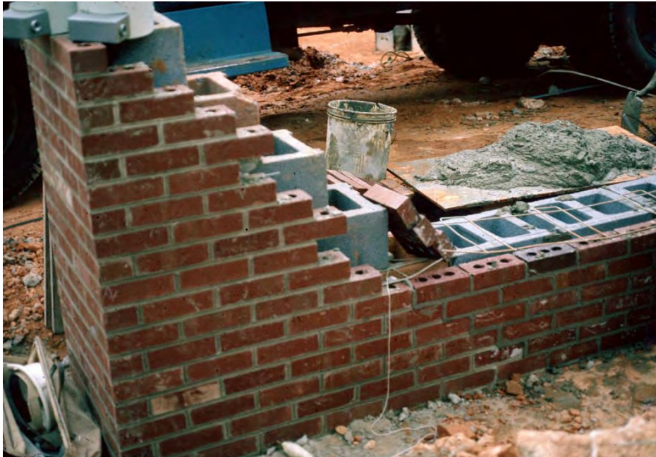
joint reinforcement adjustable veneer anchors
