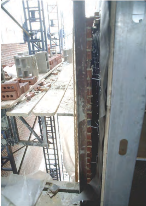
in CMU: open head joints @ 16" oc
