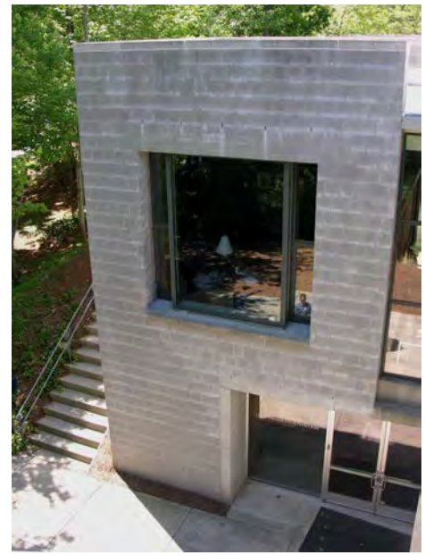
REINFORCED CONCRETE BLOCK WALLS When concrete block walls are subjected to lateral forces such as caused by wind, earth pressure below grade, and earthquakes, they may be reinforced as illustrated above.
