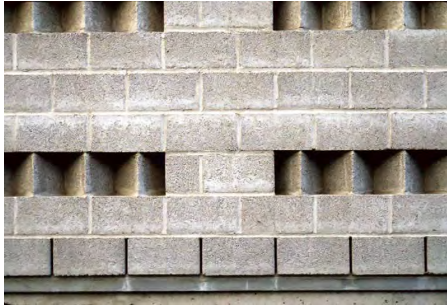
in CMU: open head joints @ 16" oc
