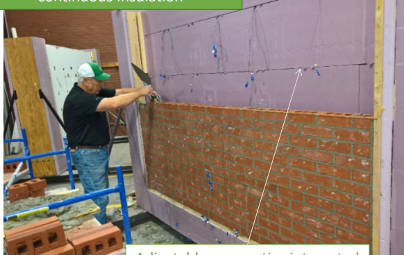
Adjustable veneer ties integrated with joint reinforcing
